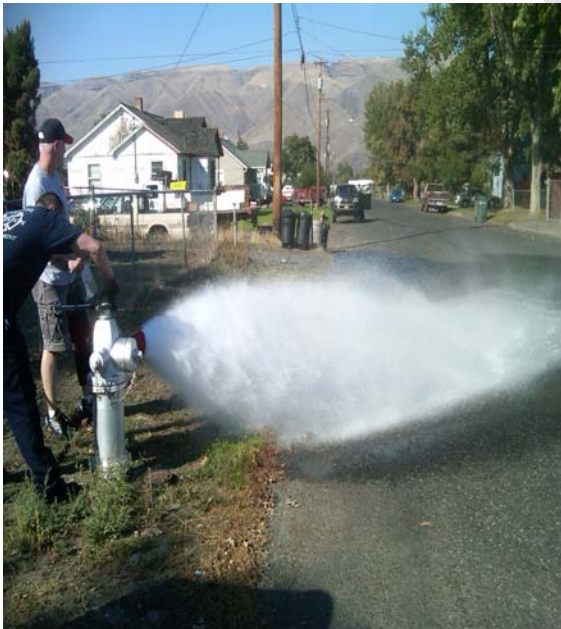
Flushing of hydrant
