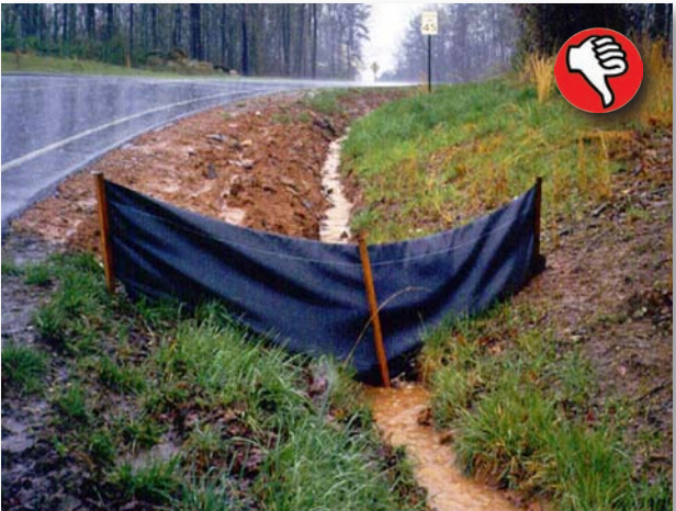
Silt fence is not an approved BMP for use as a check dam. (Source: Peter Vaughn, A3E Consultants)
