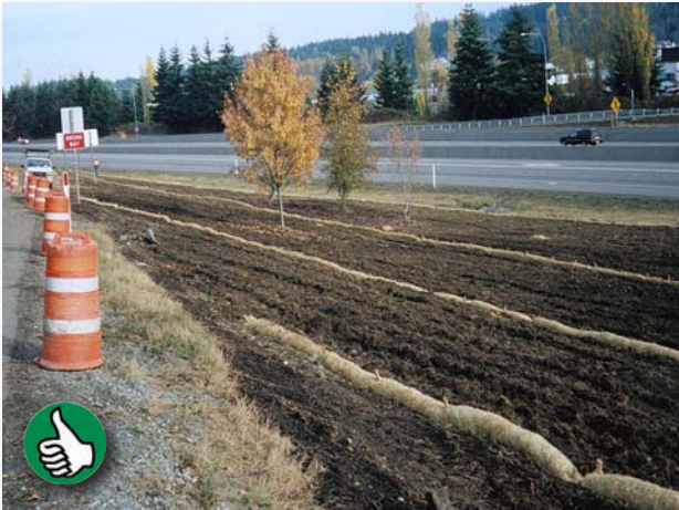
Good example of properly installed wattles.
